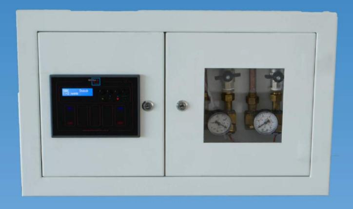
The gas control and alarm unit monitors the pressure of the compressed medical gases in the pipeline system. The gases can also be interrupted from the unit for maintenance operations or malfunctions. The pressure can be set on the LCD control screen. The unit is available for 1 up to 5 gases and can also be produced according to project.
